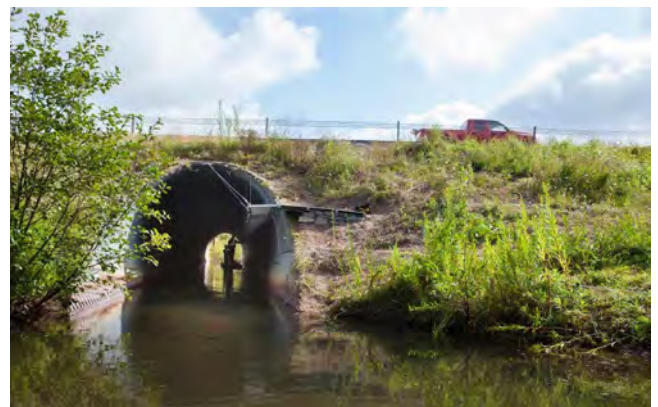
Figure 2.3.1.5: Wildlife shelf is installed in a culvert near Boonville, N.Y. Kurt Gardner/The Nature Conservancy via AP.
