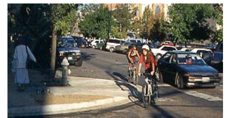
Horizontal —Bulb-out at an intersection
