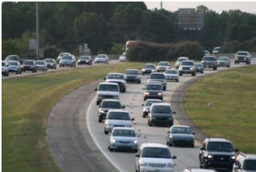
Figure 6.3.1: I-40 near US 1 Interchange
