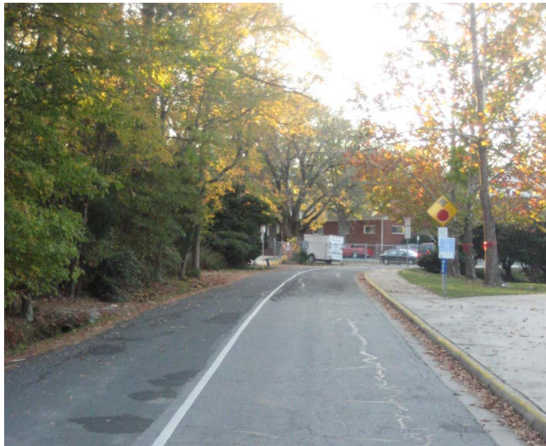
Figure 20: Pavement Markings on Shelton Street
