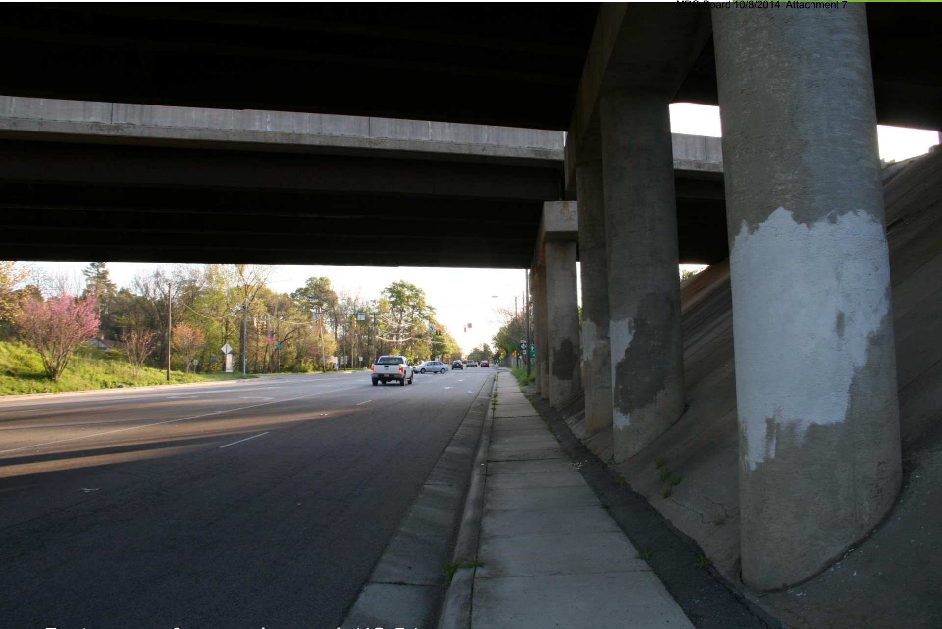
Facing east from underneath NC-54 overpass
