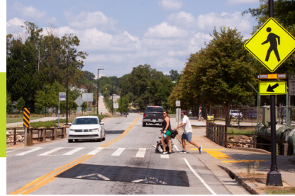
Rectangular Rapid Flashing Beacon (RRFB)
