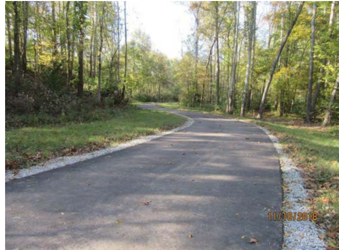
Above: Example where trees were intentionally cut to a distance of 14' from the trail pavement (Wolf River Greenway, Memphis, TN)
